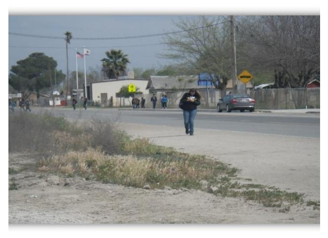
Figure 3: Avenue 54, between Lake Rd and Wilber. Sidewalk is non-existing to differentiate from roadway. Sidewalk, curb, gutter, asphalt paveout, and driveway are proposed.
