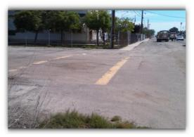
Figure 5: Sidewalk improvement proposed at Avenue 54 at Lake Road, Existing sidewalk is less than 3 feet wide and not in compliance with ADA standards.
