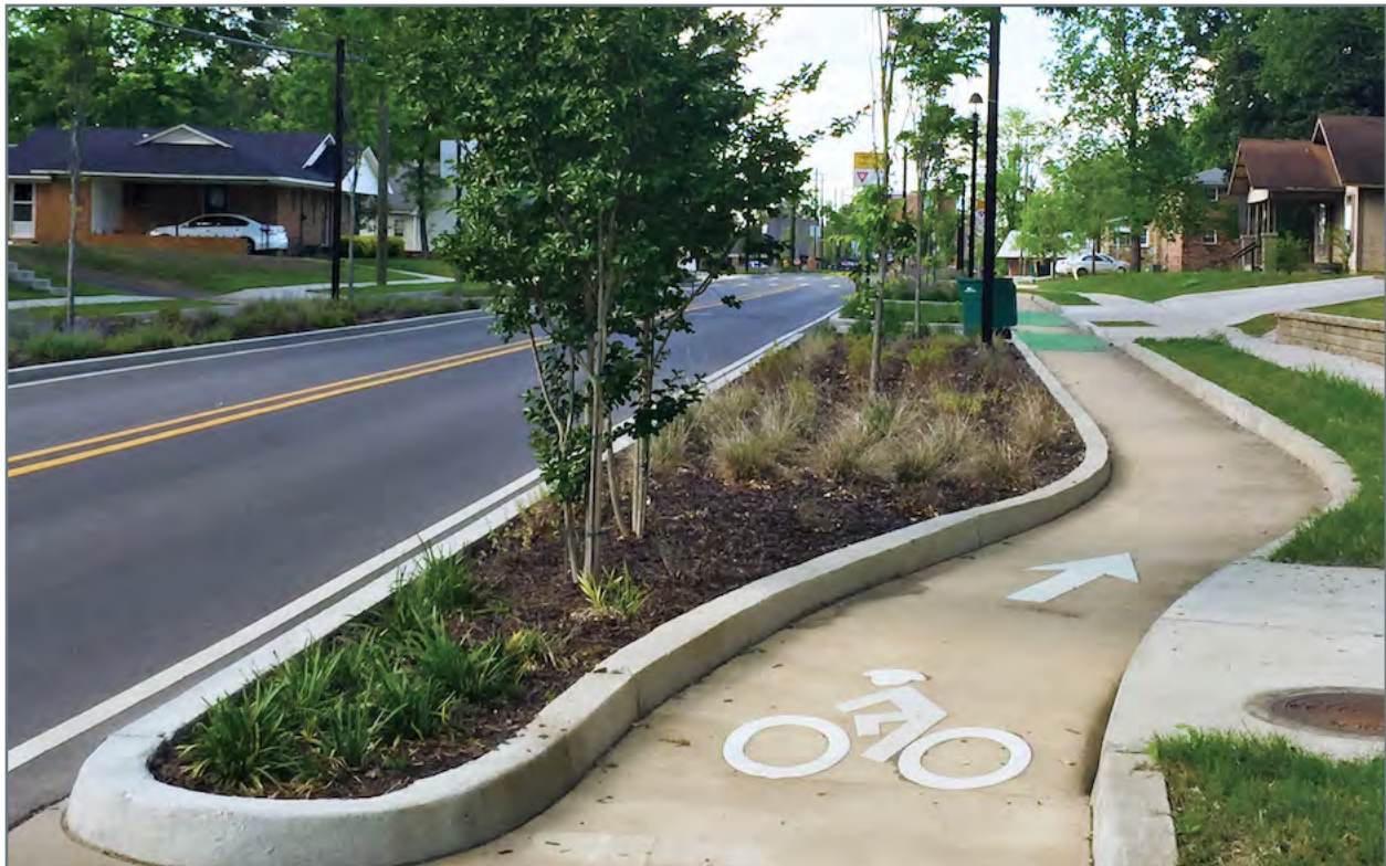
Figure 4.18 Class IV Bike Lane Protected by Curb and Landscaping
