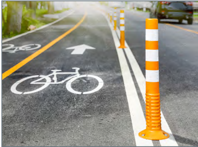
Figure 4.16 Class IV Bike Lane Protected by Flexible Bollards
