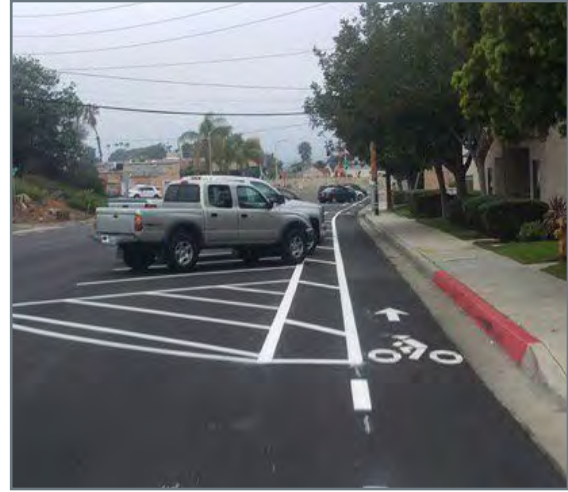
Figure 4.17 Class IV Bike Lane Protected by on-street parking
