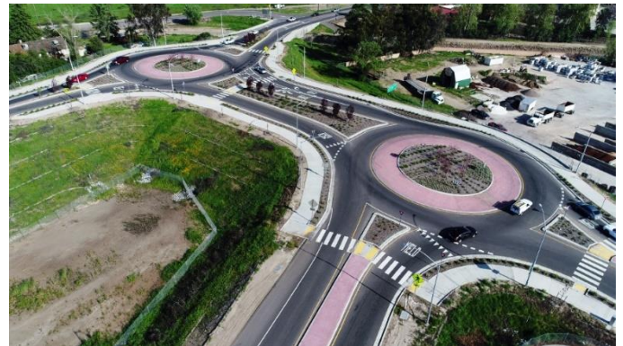
SR-198 and Farmersville Blvd Roundabouts (Farmersville, CA)
